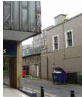
Poor servicing in Rose Street Lane
